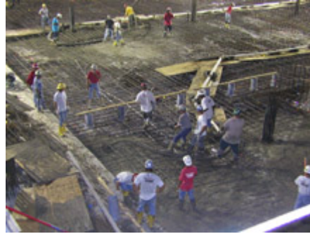
Pumps line-up and deliver 1,720 cubic yards
