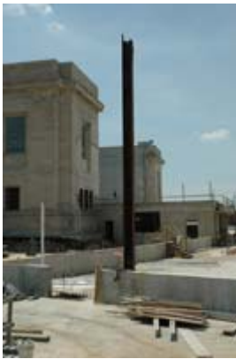
First Column in Place
