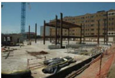
Columns, Beams, and Purlins
