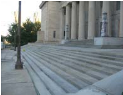
South Entrance Steps
