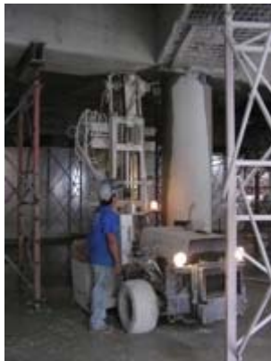
Garage Hydrodemolition
