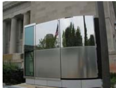
Curtainwall Mock-Up site, St. Clair St.
