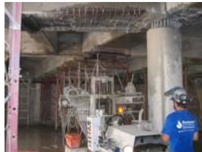
Garage Hydrodemolition
