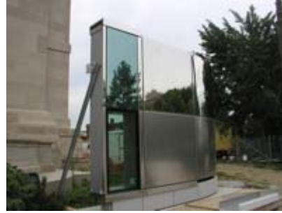
Curtainwall Mock-Up site, St. Clair St.
