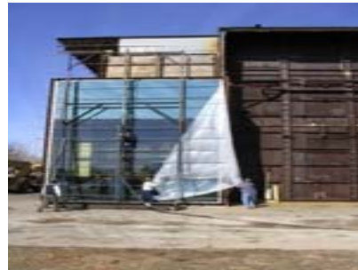
Curtainwall – large scale test site
