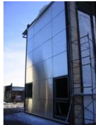
Curtainwall – large scale test site
