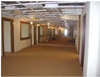
Cret - inside renovation
