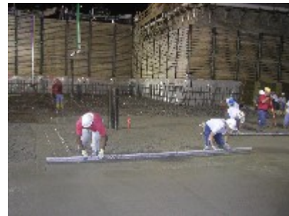
Workers, knee-high in concrete, guide the pumping tubes to position the concrete at desired locations, and level surfaces
