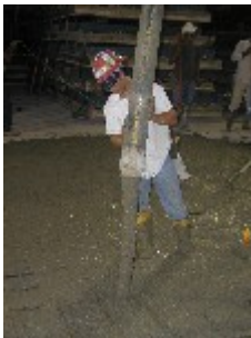
Workers, knee-high in concrete, guide the pumping tubes to position the concrete at desired locations, and level surfaces
