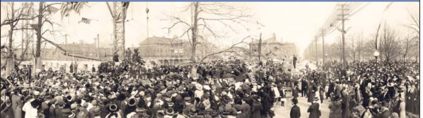
March 24, 1916 . . . the laying of the cornerstone for Central Library
